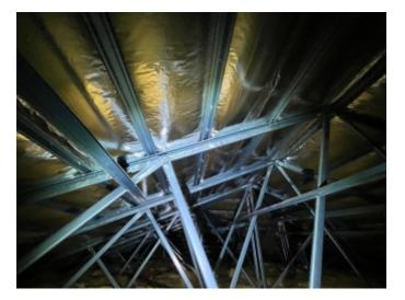
Showing example of insulation to the roof space
